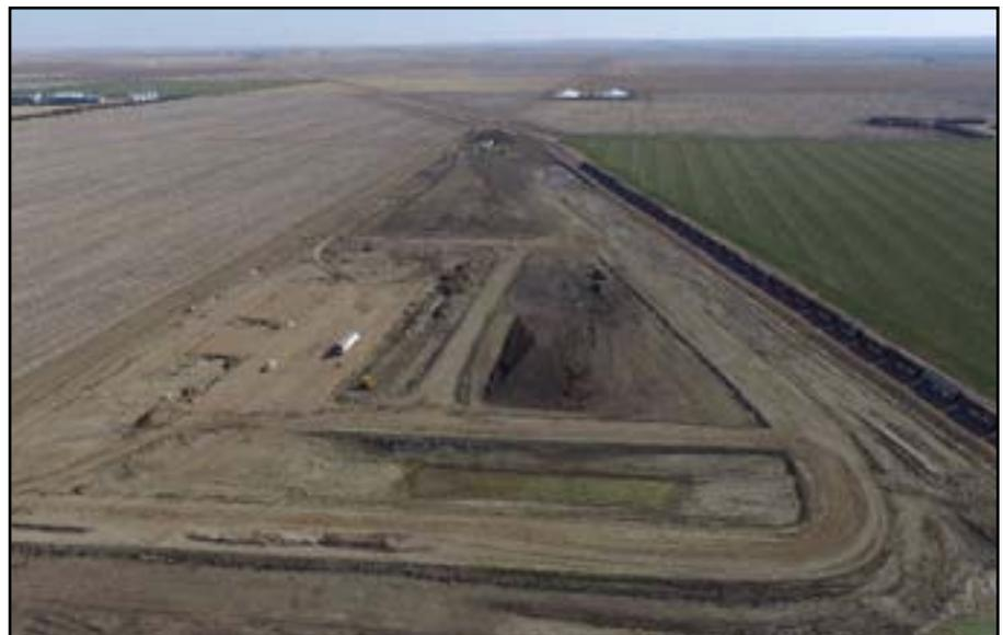
*Areas that have been filled and compacted for the base of the first structures on the Ringneck Energy site can be seen to the left in the photo. The enclosed fermentation structure will be the first constructed, as it has the most complex internal components and will take the longest to complete.*
